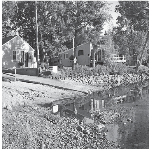
Lakeside Landing Marina at the low point of the early drawdown. Days later these buildings were surrounded by water. Alliance Photo
