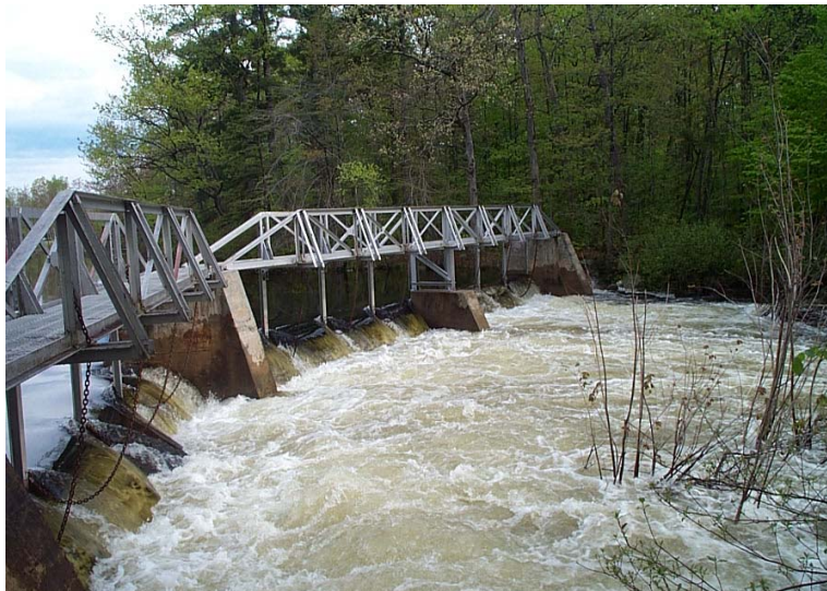
Water empties from the lake this spring after the dam gates were opened to alleviate flooding. More studies are needed to help determine how best to manage the level of the lake. Alliance Photo
